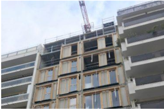
photo North by NorthWest Architectes
